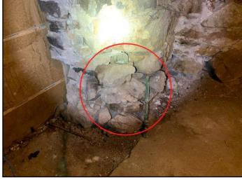
84. Spalling, crumbling or broken material
