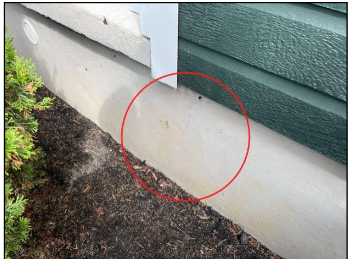
34. Parging cracked
