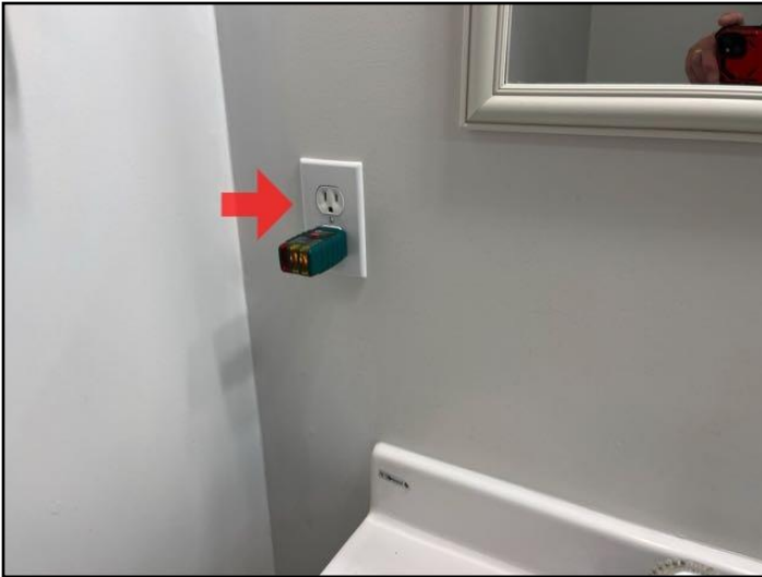
45. GFCI/GFI needed (Ground Fault Circuit...
