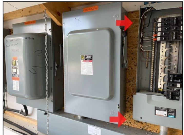
40. Inappropriate mounting surface
