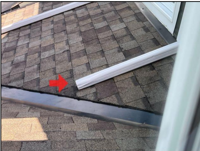
11. Discharge onto roofs
