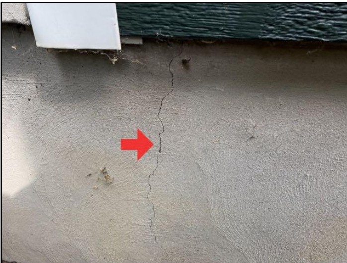
33. Parging cracked
