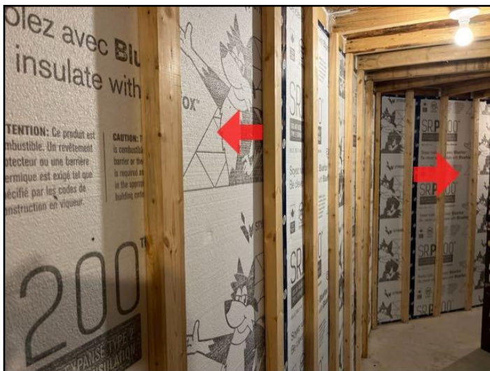
47. Exposed combustible insulation
