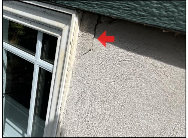
36. Parging cracked
