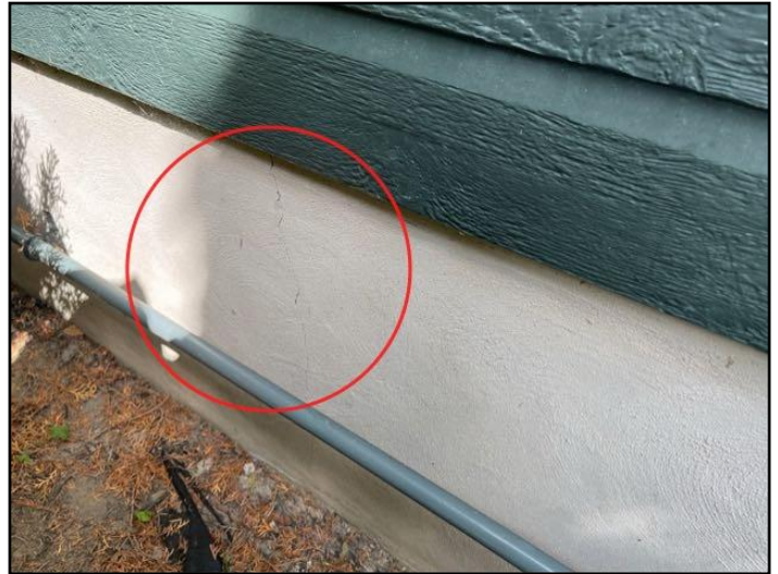
32. Parging cracked
