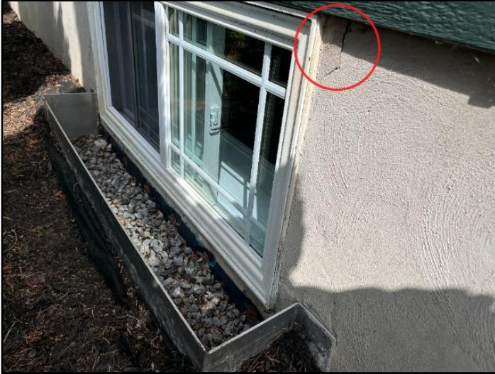
35. Parging cracked
