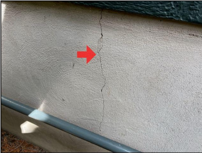
31. Parging cracked
