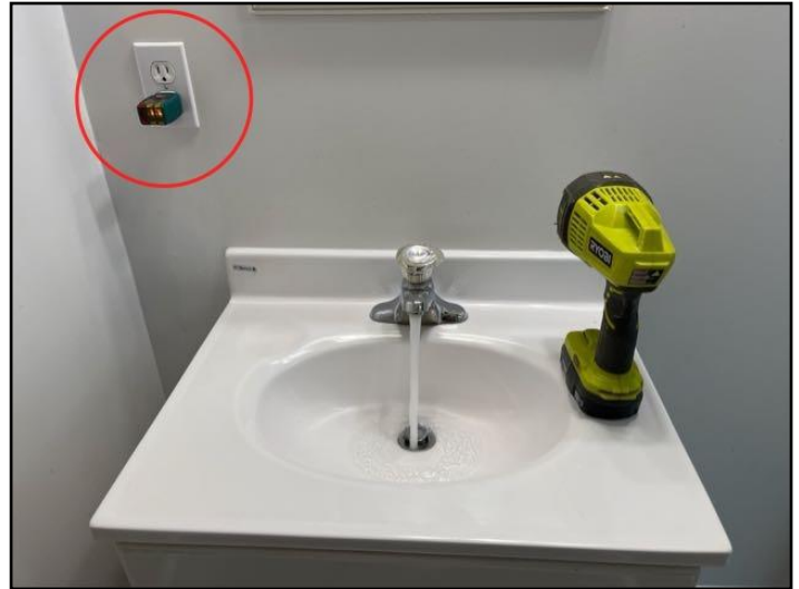
46. GFCI/GFI needed (Ground Fault Circuit...
