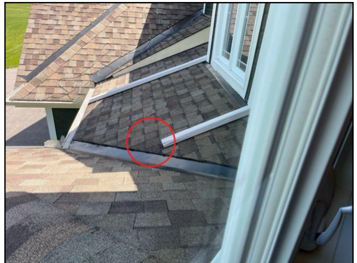
12. Discharge onto roofs
