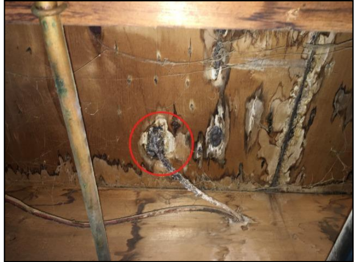
54. Electrical wiring in damp area
