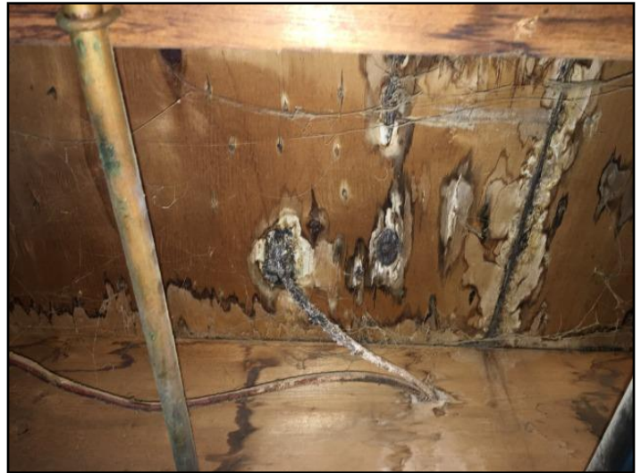
47. Rot/Water damage
