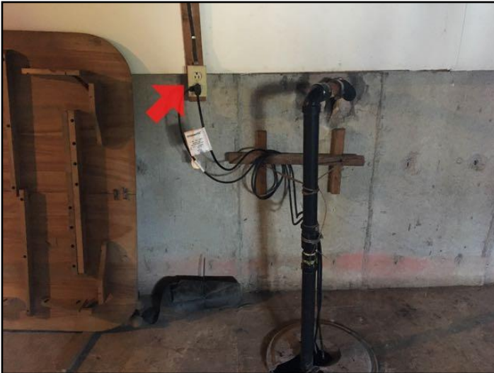
61. No GFCI/GFI (Ground Fault Circuit...
