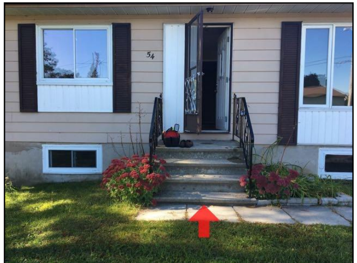
40. Trip hazards/Step not uniform
