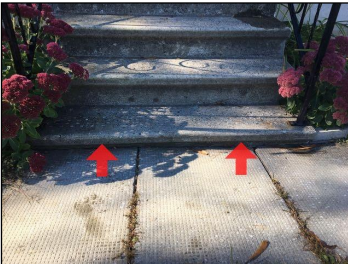
39. Trip hazards/Step not uniform
