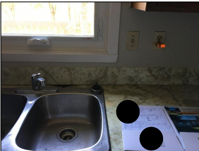
59. GFCI/GFI needed (Ground Fault Circuit...
