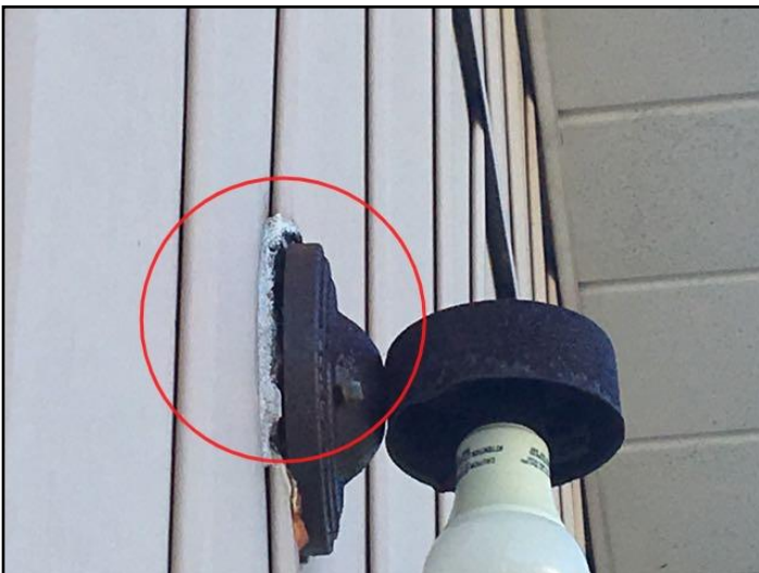
15. Caulking - deteriorated, loose or missing
