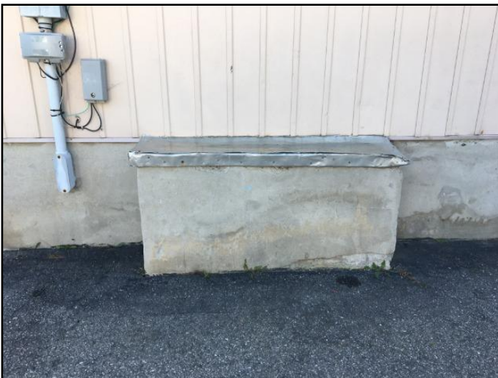
19. Caulking missing or deteriorated
