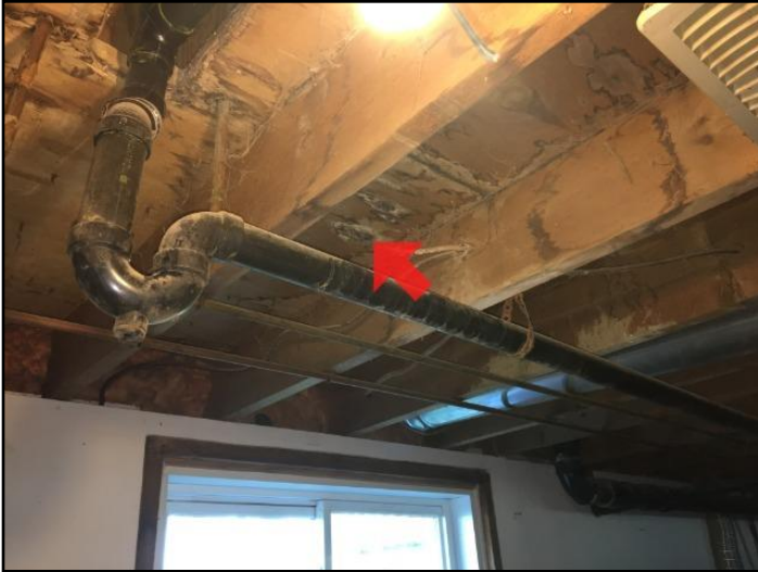
53. Electrical wiring in damp area
