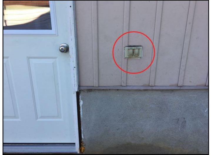
22. Caulking missing, deteriorated or loose
