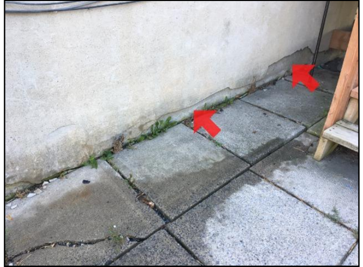
26. Parging damaged or missing
