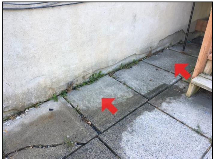
42. Improper slope or drainage
