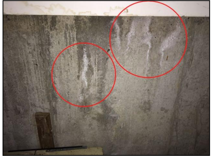
80. Efflorescence
