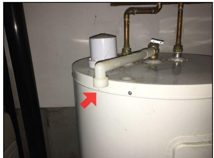
68. Discharge tube missing
