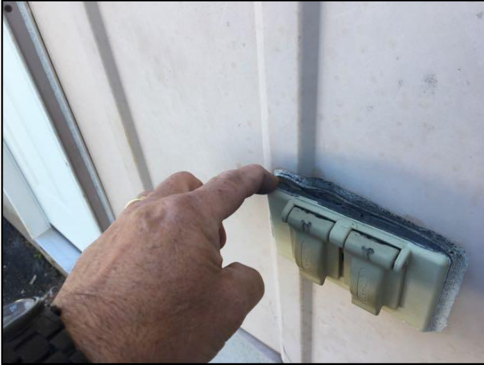
21. Caulking missing, deteriorated or loose
