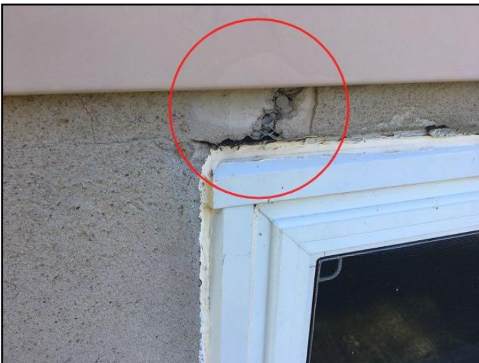
23. Parging missing/deteriorated
