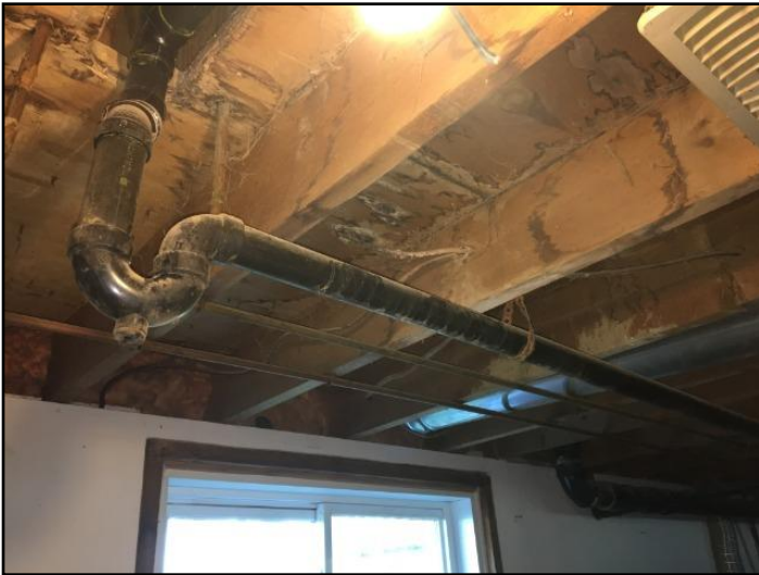
46. Rot/Water damage
