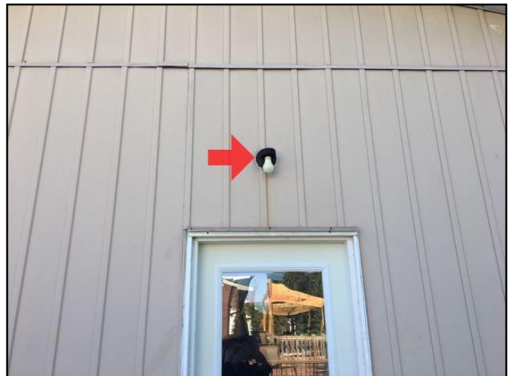
16. Caulking - deteriorated, loose or missing
