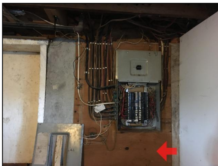
52. Inappropriate mounting surface
