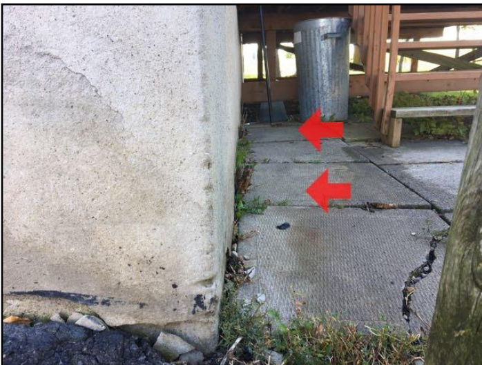
41. Improper slope or drainage
