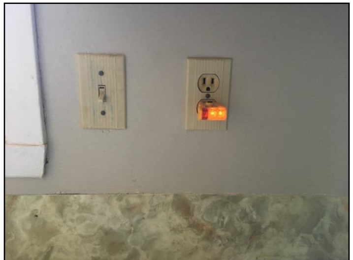
60. GFCI/GFI needed (Ground Fault Circuit...
