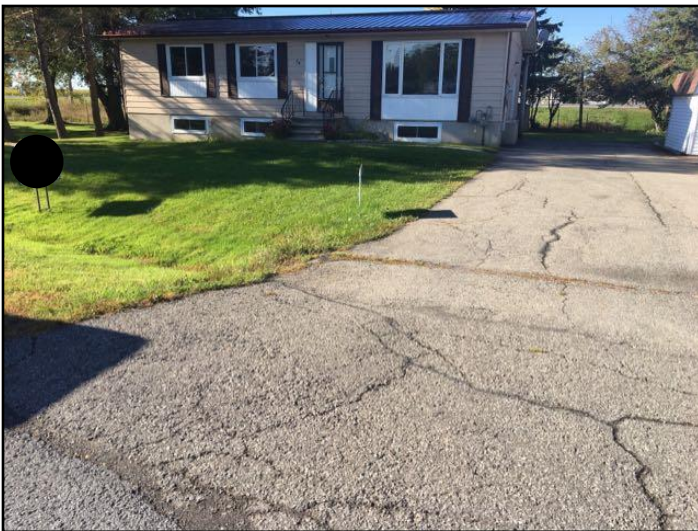
44. Cracked or damaged surfaces
