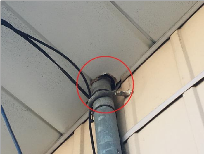
17. Caulking missing or deteriorated
