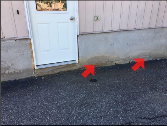
25. Parging damaged or missing
