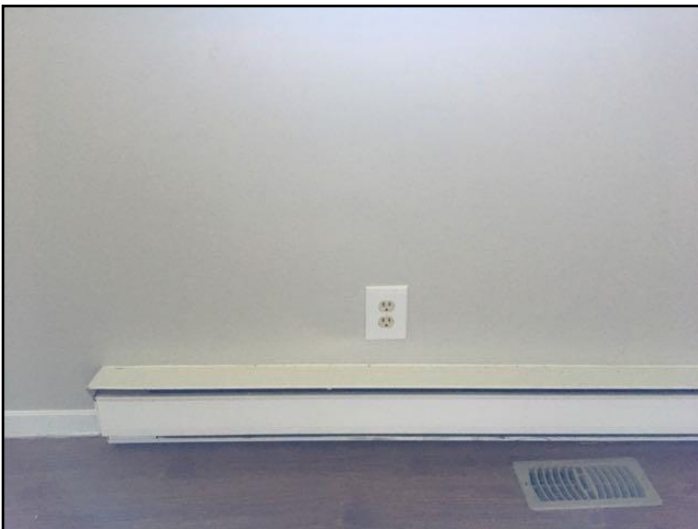
63. Receptacle poor location
