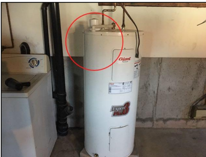
67. Discharge tube missing
