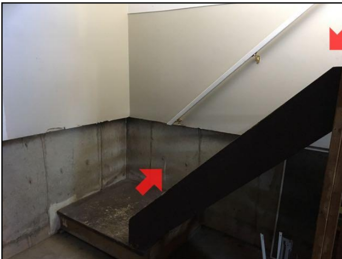
77. Missing guardrail
