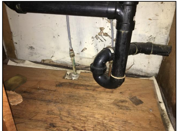
73. Water damage
