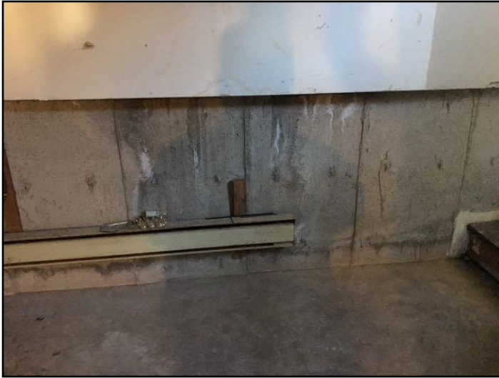
79. Efflorescence
