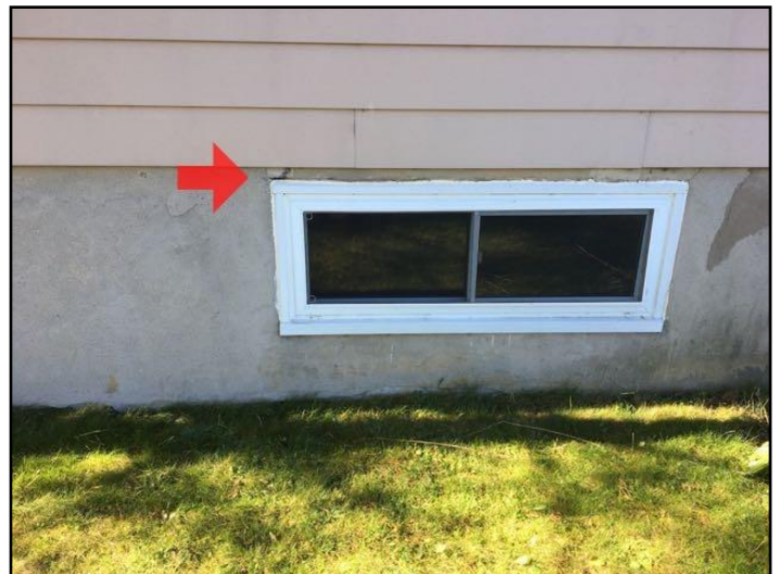
24. Parging missing/deteriorated
