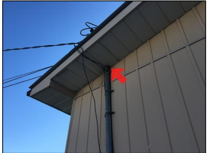
18. Caulking missing or deteriorated
